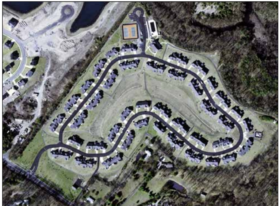
As seen in this aerial view from 2002, the homes were in place after the land had been contoured, but many trees were yet to be planted.
